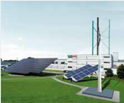
Energy solutions Park, Bielefeld, Germany
