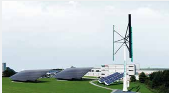
Energy solutions park, Bielefeld, Germany
