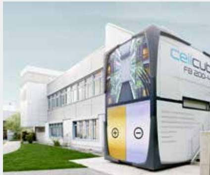
Energy solutions Park, Bielefeld, Germany
